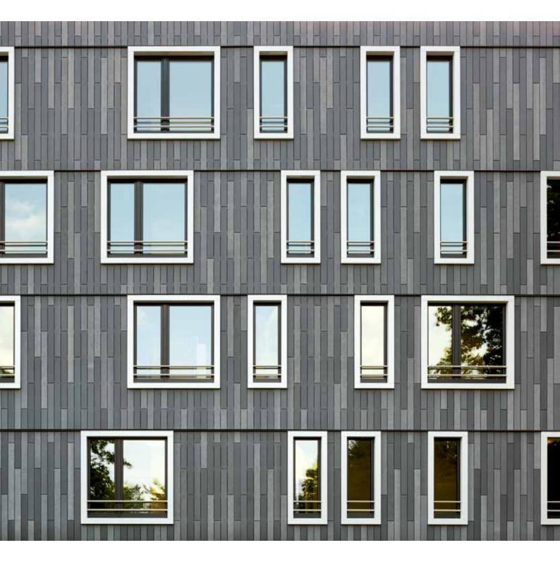
Besides the flexible use of the building, the modular construction system of the student's residential complex also scored with extremely short construction periods and top execution quality. The high level of architectonic detailed engineering, prefabrication of system components and the use of pre-assembled bathroom modules contributed to the success of this building complex, even in terms of economic aspects.
